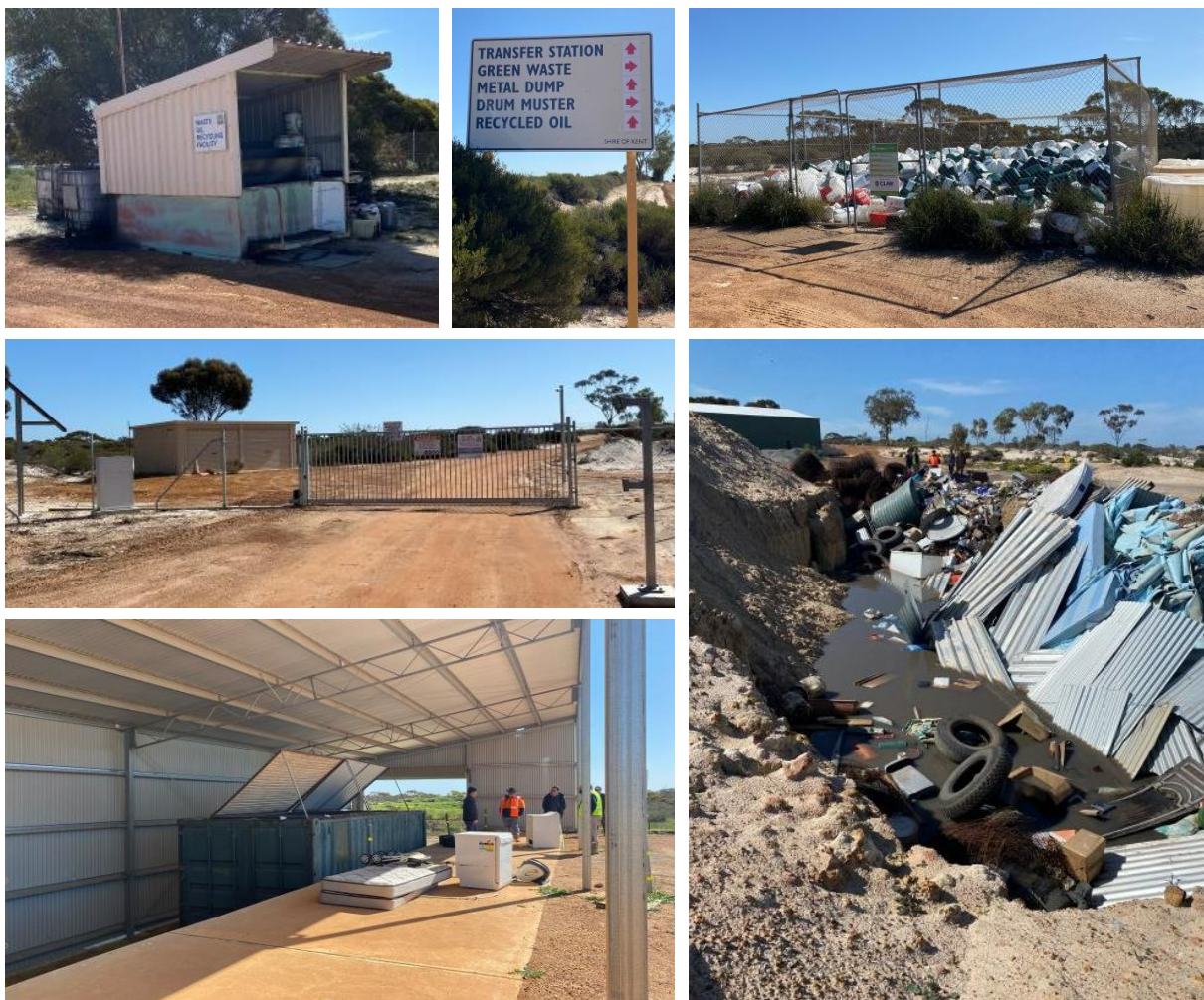
Figure 3.5 Pingrup waste facility infrastructure
